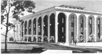
Richland County Courthouse
